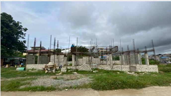
CONSTRUCTION OF TWO STOREY COLLEGE OF VETERINARY BUILDING
