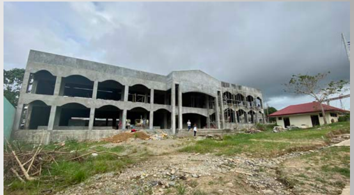
CONSTRUCTION OF TWO-STOREY INFORMATION TECHNOLOGY COMPLEX
