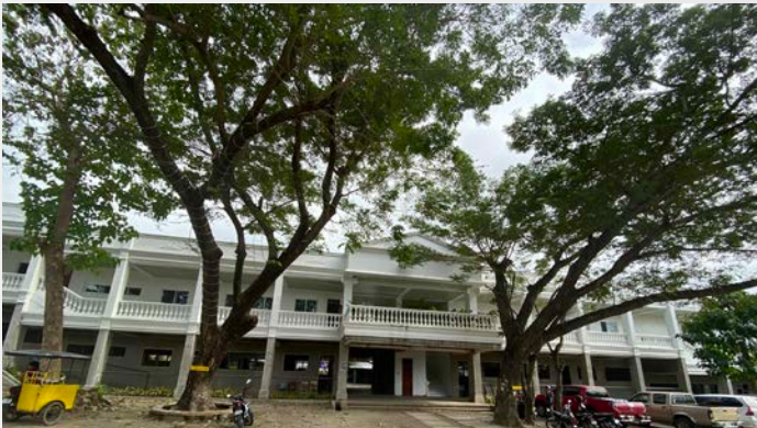
CONSTRUCTION OF SECOND FLOOR COLLEGE OF PUBLIC ADMINISTRATION BUILDING C
