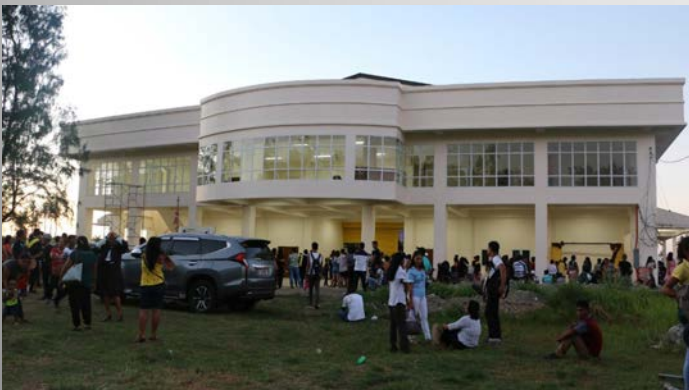
COMPLETION OF MULTI-PURPOSE GYMNASIUM (GYMPLEX)
