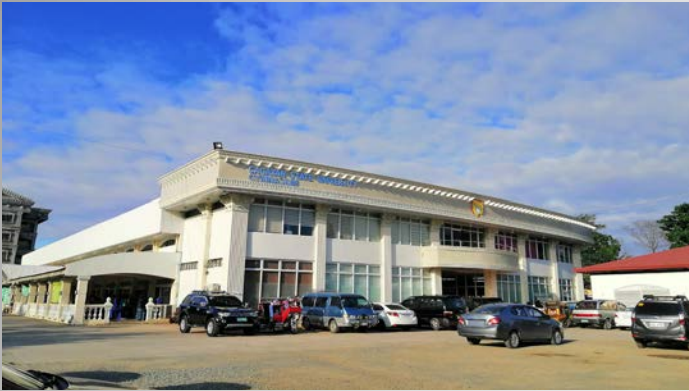
COMPLETION OF MULTI-PURPOSE GYMNASIUM
