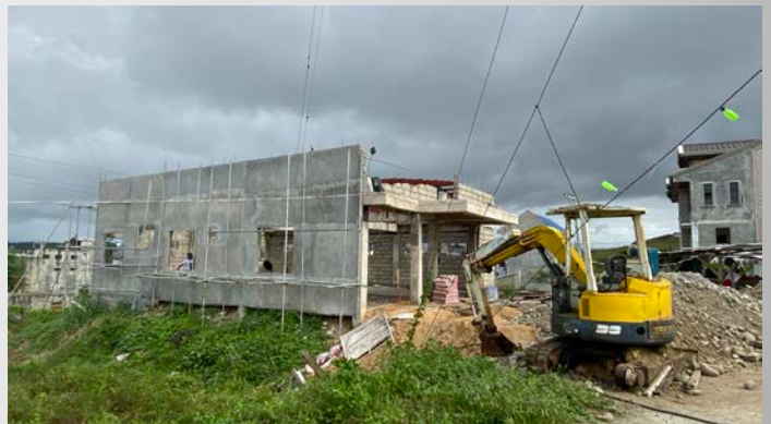
CONSTRUCTION OF LABORATORY ANIMAL FACILITY
