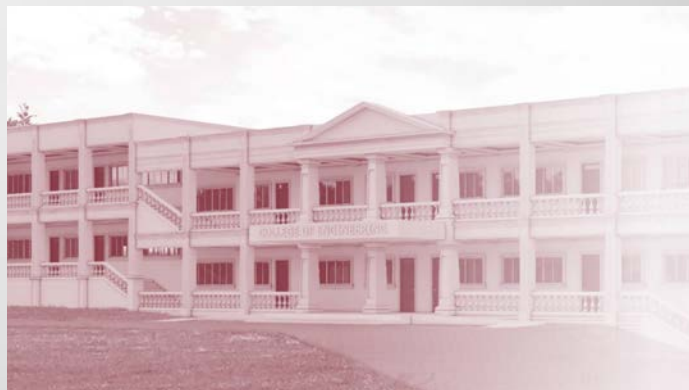
CONSTRUCTION OF SECOND FLOOR COLLEGE OF ENGINEERING BUILDING-A
