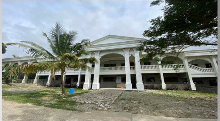
CONSTRUCTION OF SECOND FLOOR COLLEGE OF ARTS & SCIENCES BUILDING A
