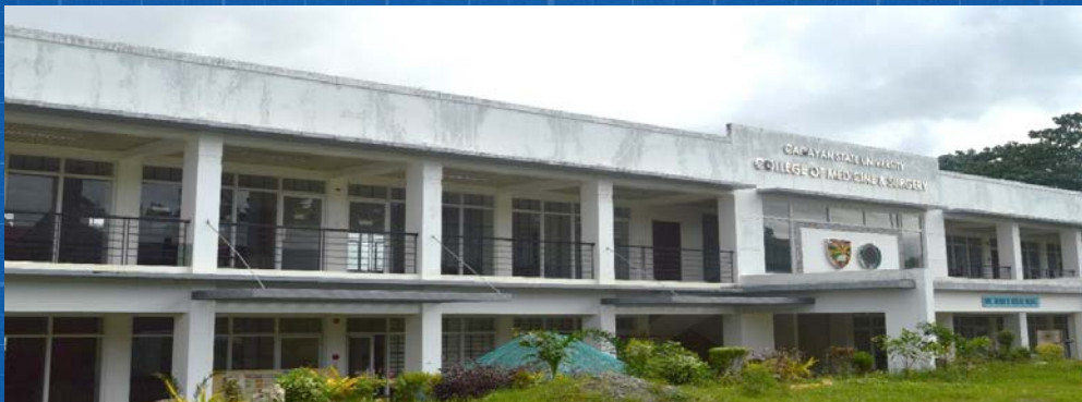
REHABILITATION OF COLLEGE OF MEDICINE NEW BUILDING Percentage Completed: 100%
