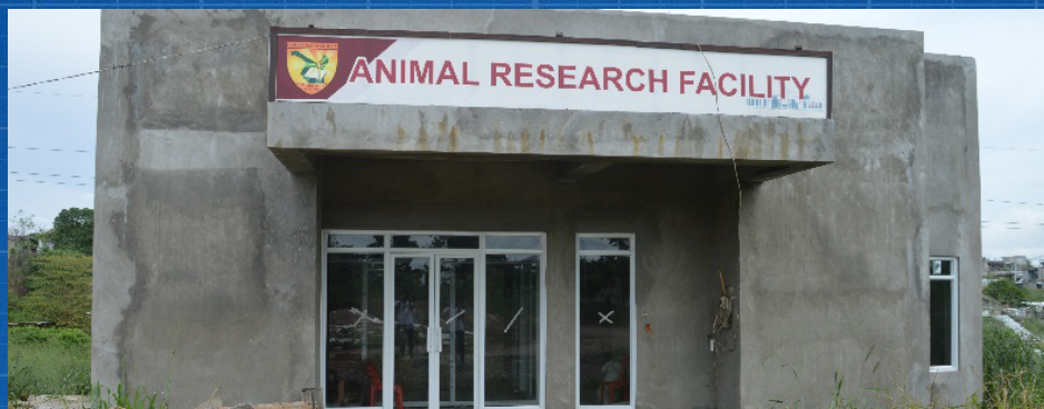
CONSTRUCTION OF ANIMAL LABORATORY FACILITY Percentage Completed: 100%
