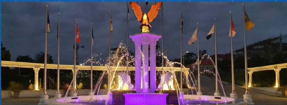
CONSTRUCTION, ROAD AND FINISHING OF CAMPUS ROTUNDA Percentage Completed: 100%
