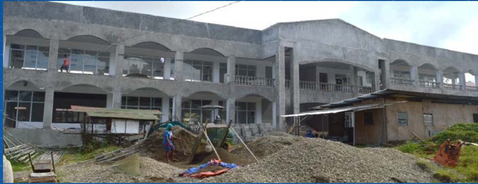
CONSTRUCTION OF INFORMATION TECHNOLOGY COMPLEX BUILDING (PHASE 1) Percentage Completed: 100%
