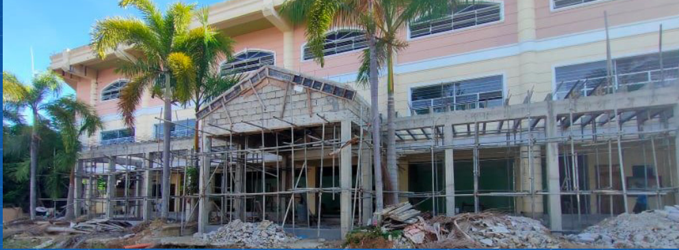
CONSTRUCTION OF CAMPUS BUSINESS CENTER Percentage Completed: 58%
