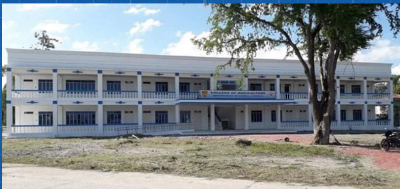
REHABILITATION OF CSU PIAT COLLEGE OF AGRICULTURE BUILDING Percentage Completed: 100%
