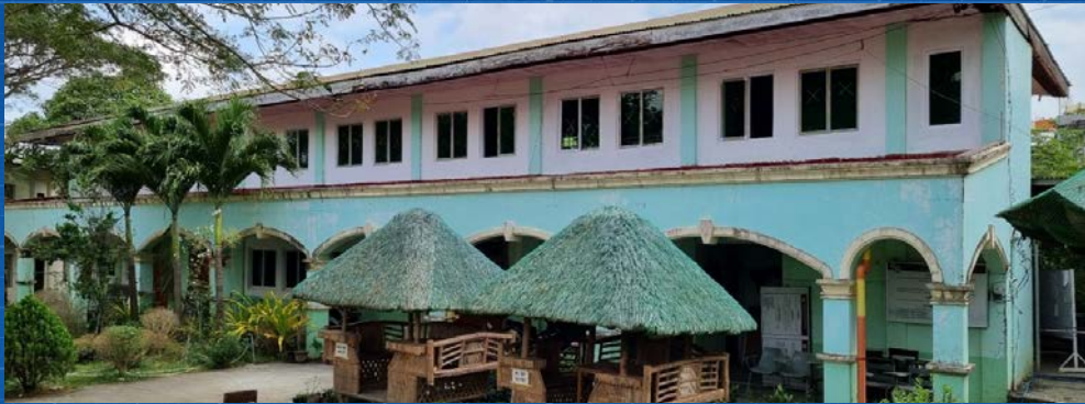
REHABILITATION OF COLLEGE OF VETERINARY MEDICINE BUILDING Percentage Completed: 100%
