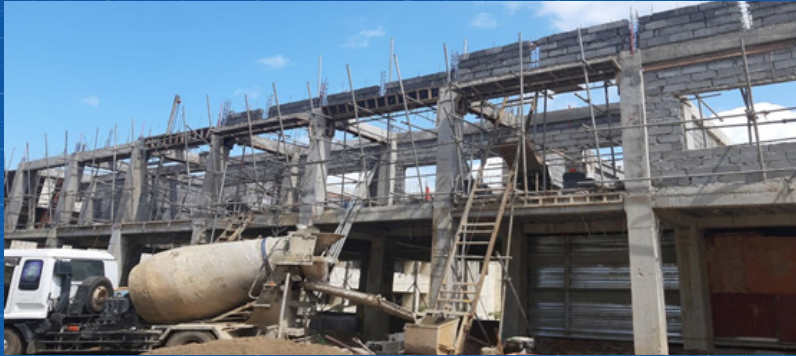
REHABILITATION OF 2-STORY ACADEMIC AND LABORATORY BUILDING Percentage Completed: 58.07%
