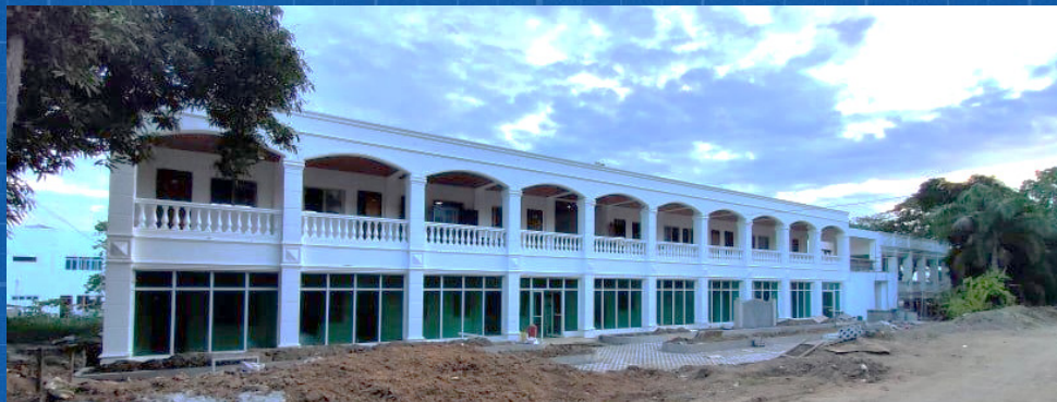
REHABILITATION OF DOST – FOOD INNOVATION CENTER BUILDING Percentage Completed: 80%
