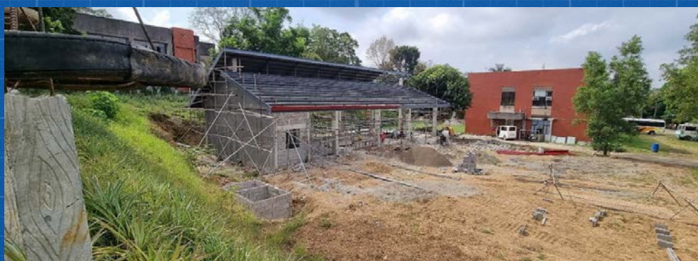
CONSTRUCTION OF CAMPUS MOTORPOOL Percentage Completed: 100%
