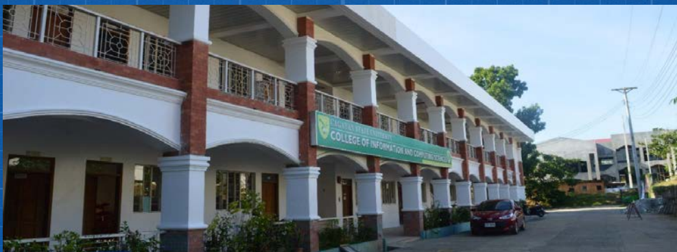
REHABILITATION OF COLLEGE OF INFORMATION & COMPUTING SCIENCES BUILDING Percentage Completed: 100%
