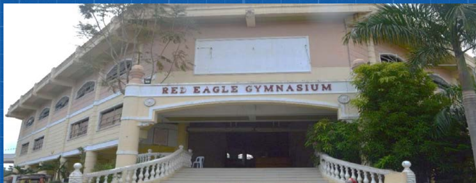
REHABILITATION OF CAMPUS GYMNASIUM Percentage Completed: 55%
