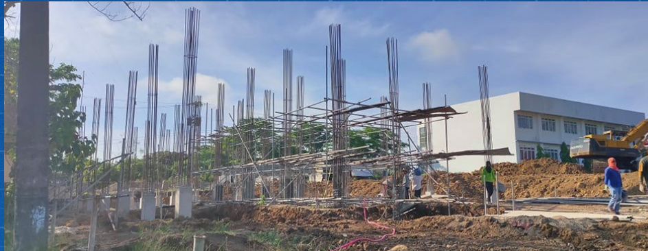
CONSTRUCTION NEW CAMPUS DORMITORY (PHASE 1) Percentage Completed: 10%
