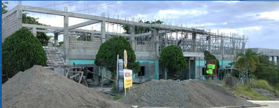
REHABILITATION OF COLLEGE OF INDUSTRIAL TECHNOLOGY BUILDING A Percentage Completed: 51%
