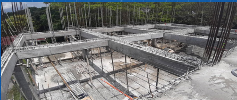
CONSTRUCTION OF 2-STORY ACADEMIC AND LABORATORY BUILDING Percentage Completed: 56.02%
