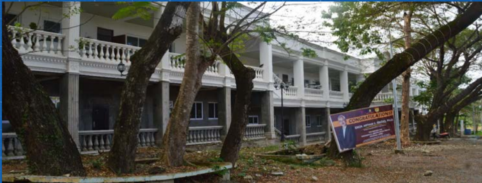
CONSTRUCTION OF COLLEGE OF PUBLIC ADMINISTRATION BUILDING C Percentage Completed: 100%
