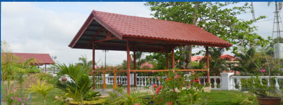
CONSTRUCTION OF TWO UNITS KIOSK Percentage Completed: 100%
