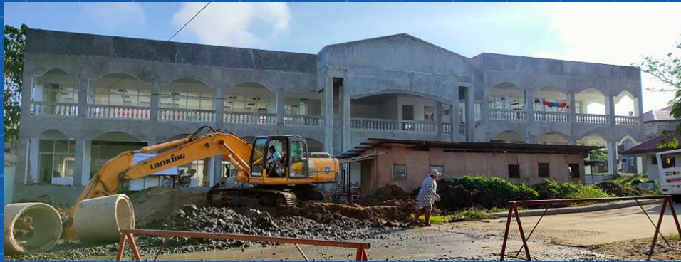
CONSTRUCTION OF INFORMATION TECHNOLOGY COMPLEX BUILDING (PHASE 2) Percentage Completed: 30%
