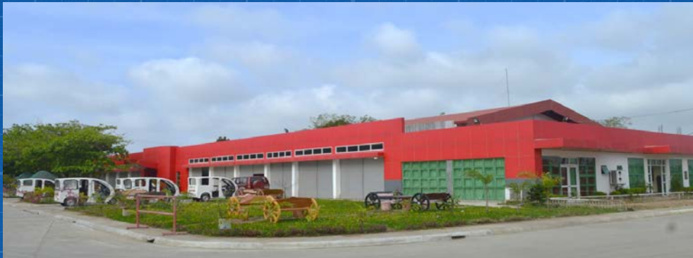
REHABILITATION OF CIT WORKSHOP BUILDING & GROUNDS IMPROVEMENTS Percentage Completed: 100%
