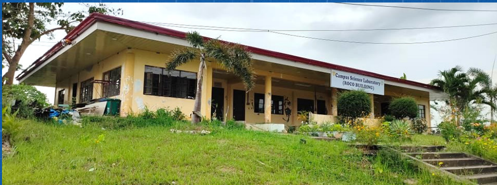
REHABILITATION OF ROCO BUILDING Percentage Completed: 100%
