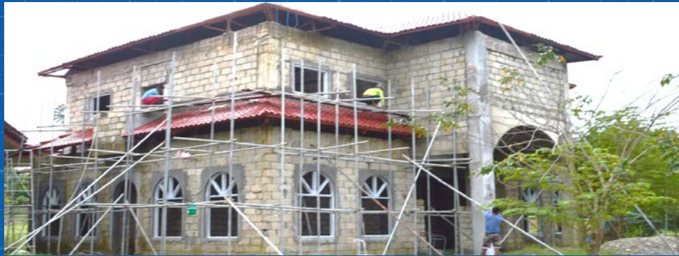
CONSTRUCTION OF RESIDENCE HALL (PHASE 1) Percentage Completed: 85%
