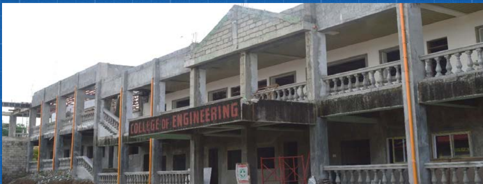
CONSTRUCTION OF COLLEGE OF ENGINEERING BUILDING A Percentage Completed: 70%
