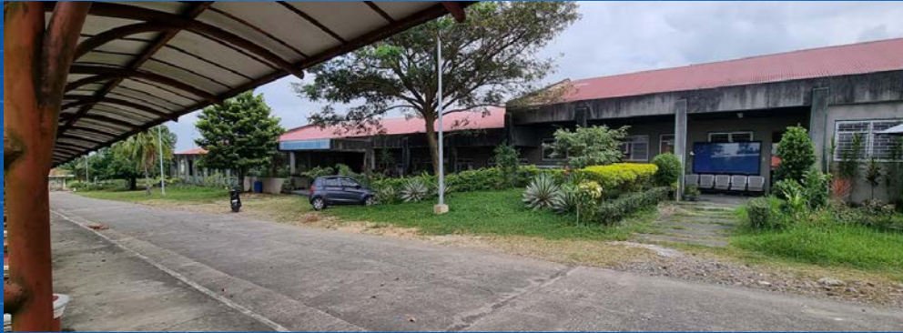
REHABILITATION OF COLLEGE OF MEDICINE & SURGERY OLD BUILDING Percentage Completed: 100%
