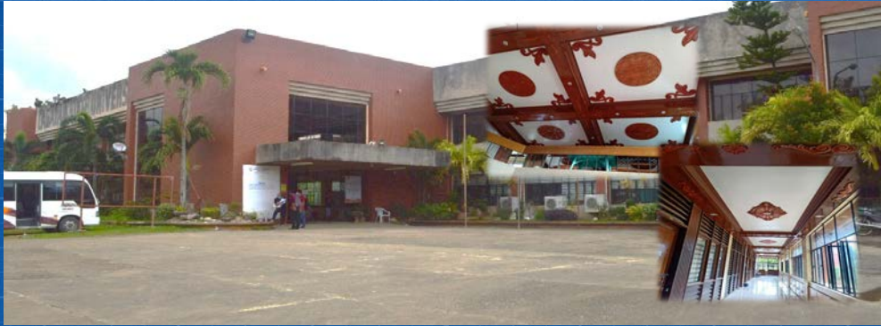
REHABILITATION OF CAMPUS ADMINISTRATION BUILDING Percentage Completed: 100%
