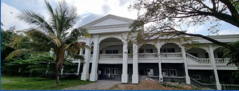
CONSTRUCTION OF COLLEGE OF ARTS & SCIENCES BUILDING A Percentage Completed: 100%
