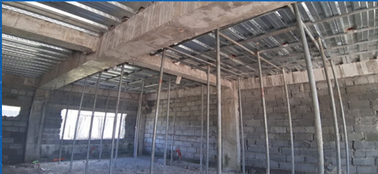
CONSTRUCTION OF 2-STORY ACADEMIC AND LABORATORY BUILDING Percentage Completed: 55.09%
