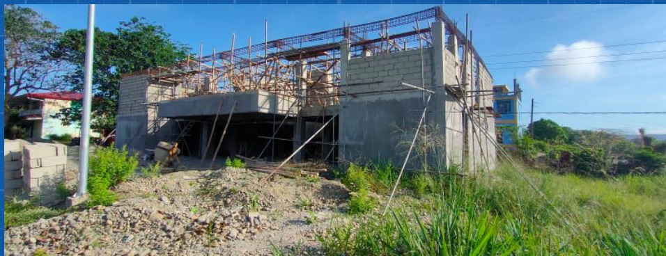
CONSTRUCTION OF TWO STOREY VETERINARY MEDICINE BUILDING Percentage Completed: 70%
